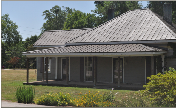
Figure 11. The Yarbrough House sits across from City Hall and within the future Town Center. The City plans to establish a welcome/history/arts center and coffee shop there.
