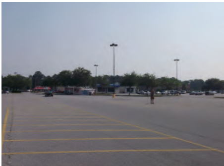
Existing parking lot island consists of only painted yellow stripes
