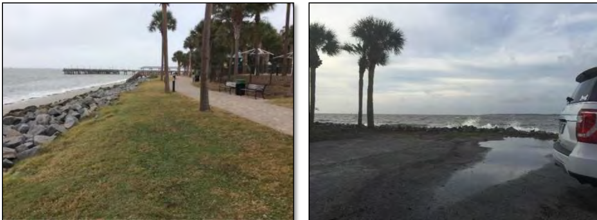
Figure 5.11: Photos of Johnson Rocks at Neptune Park (left, low tide; right, high tide)
