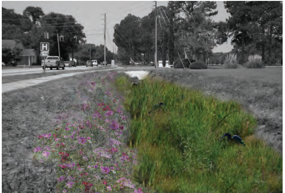
Improvements to the bioswale along Fourth Street
