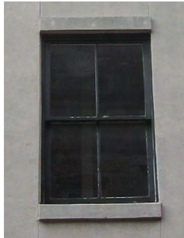
Stucco Header and Sill
