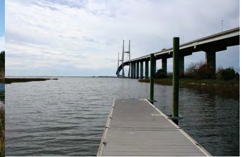
View from floating dock Sidney Lanier Bridge.
