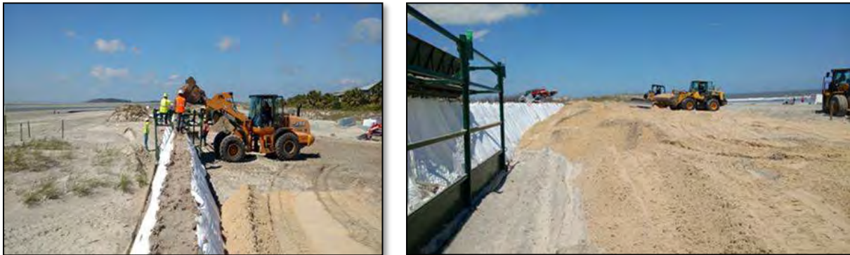
Figure 2.3: PermaShield™ being installed at 19th St on Tybee Island. Photo Credit: Guardian Retention Systems
