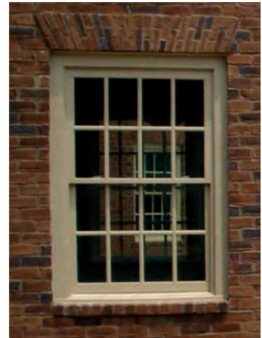
Brick Header and Sill
