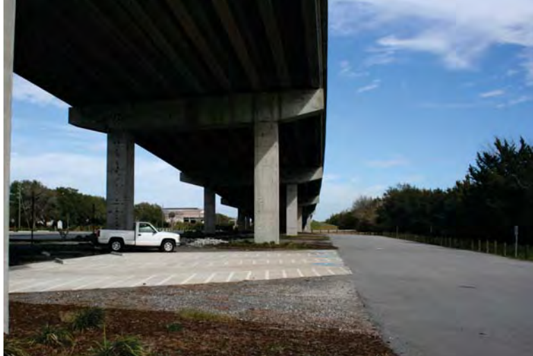
View looking North following overpass.
