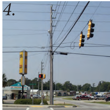
2. Streetscape, signage, and curb cuts along Altama Avenue 3. Altama Avenue center median near intersection with Community Road 4. Typical string mounted traffic signals
