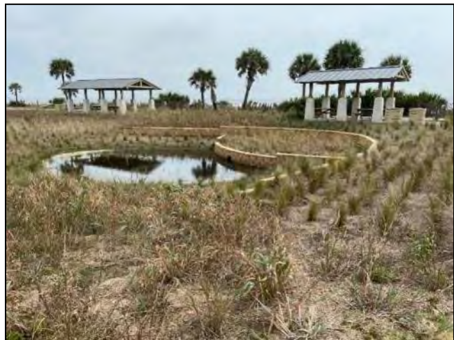
Figure 5.10: Oceanview Beach Park GI/LID Practices – Bioretention with Pervious Concrete Border (left) and Constructed Stormwater Wetland (right).
