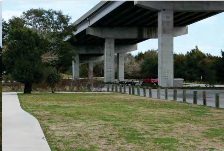
Existing green space with protective bollards.
