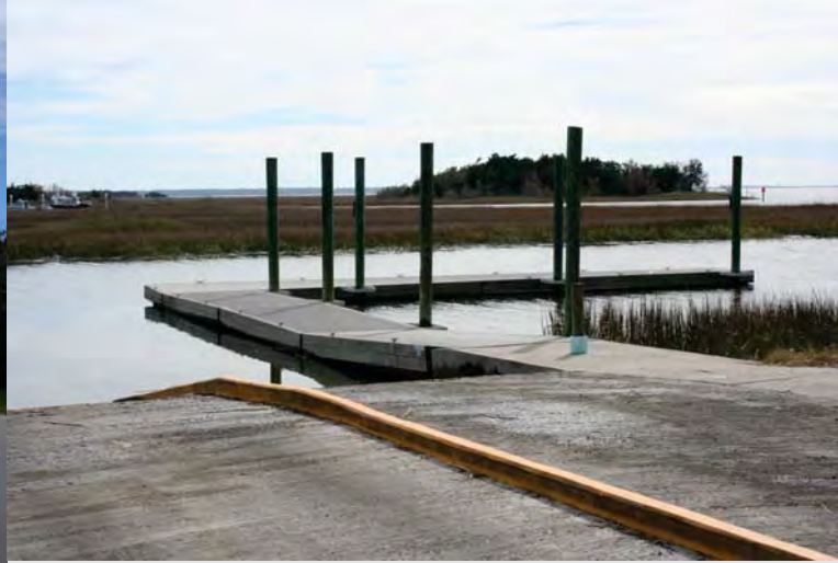
View of existing floating dock and boat ramp.
