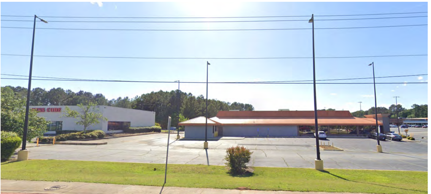
Figures 128 & 129: Underutilized business on SR-85 (above) and Merchants Square on SR-85 (below)
