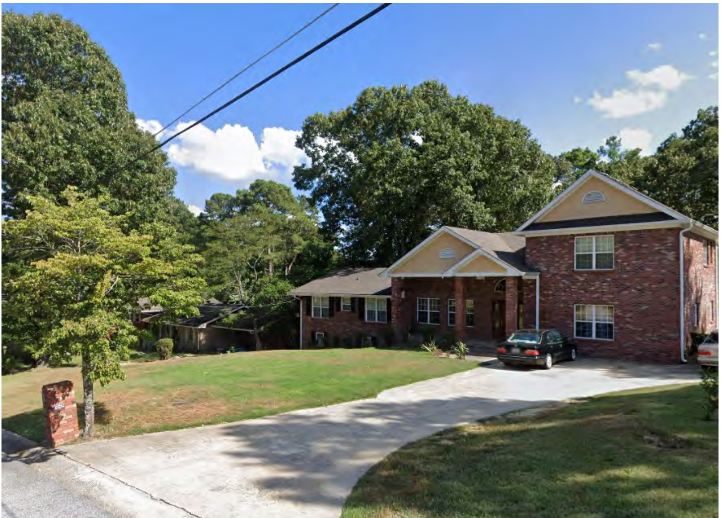
Figure 152 : Suburban House in City of Riverdale, GA
