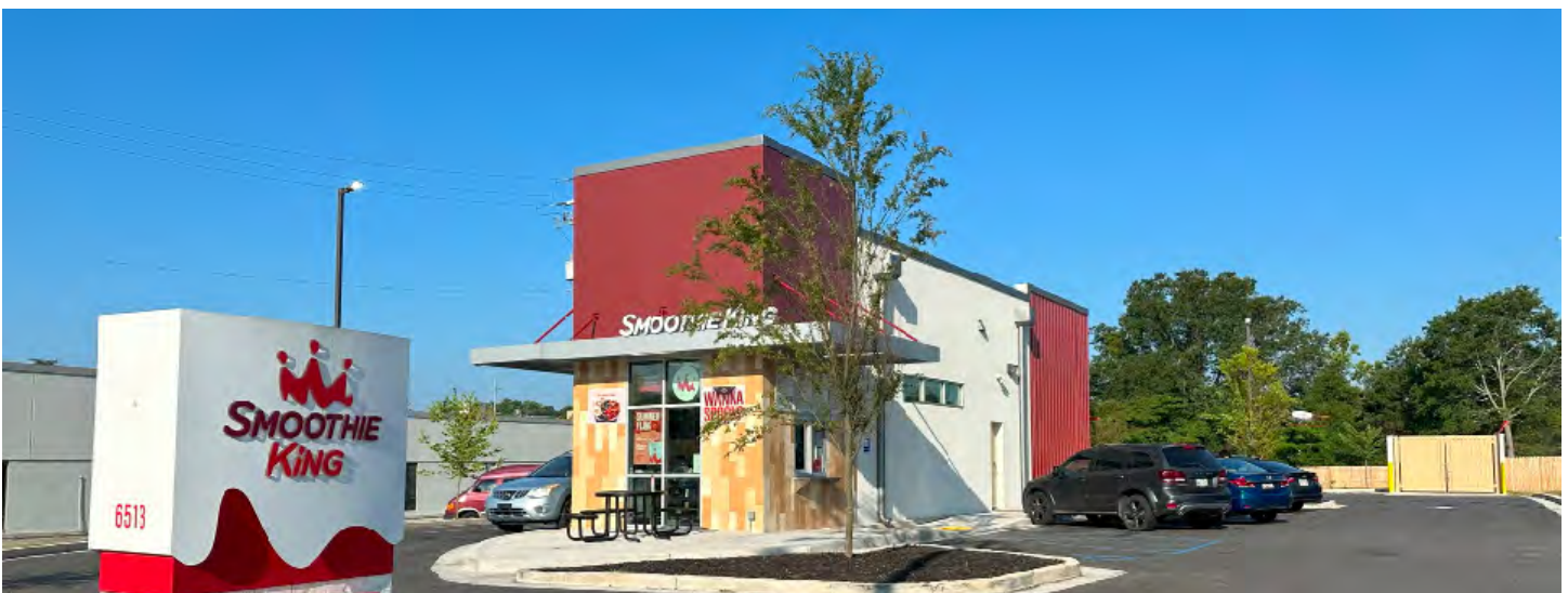
Figure 61: Smoothie King in Riverdale along SR- 85
