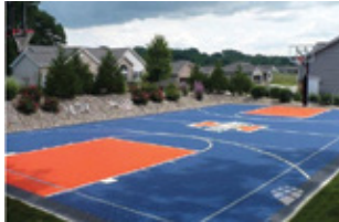
⑧ Refurbished Basketball Court
