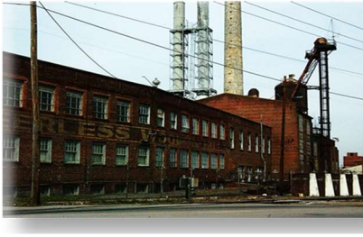
Figure 58. Abandoned Peerless Mill, Rossville
