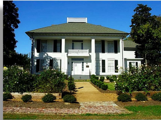
Figure 74: Historic Marsh House
