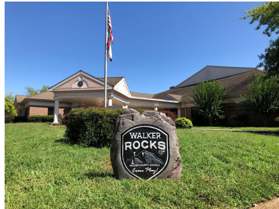
Figure 38. Walker Civic Center Campus at U.S. 27, Rock Spring, Ga.
