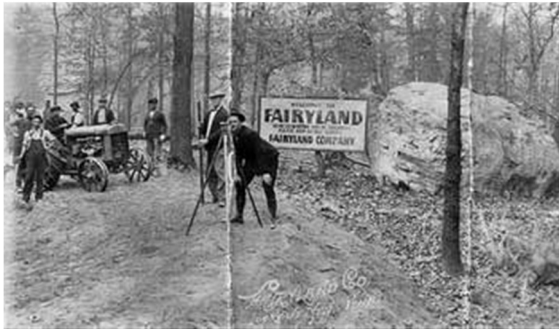
Figure 12. Surveying the Fairyland Club - https://lookoutmountain.club/HistoryOfFairylandClub
