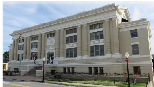
Figure 5. 1918 Historic Courthouse in LaFayette
