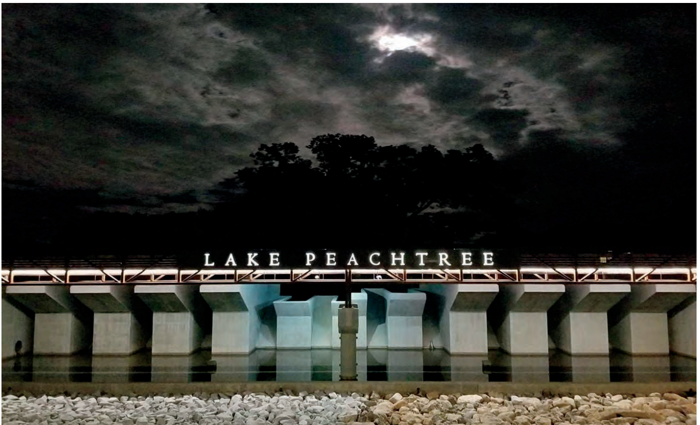
The Peachtree City Spillway is a significant infrastructure investment
