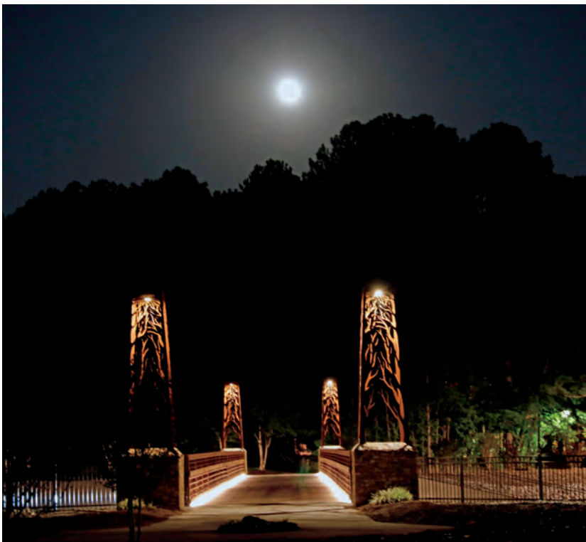
The Lake Peachtree Spillway and Path Bridge is an important capital improvement in Peachtree City.
