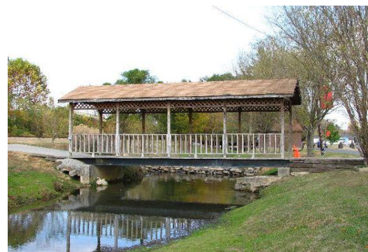
Figure 24: Walking Bridge in Dowdy Park. City of Summerville, GA
