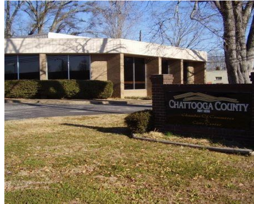
Figure 23: Chattooga County Chamber of Commerce and Civic Center. Photo courtesy of the Chattooga Chamber of Commerce
