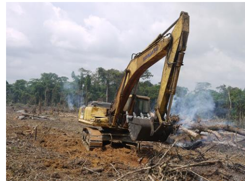
Figure 32: Example of Infrastructure expansion on construction site
