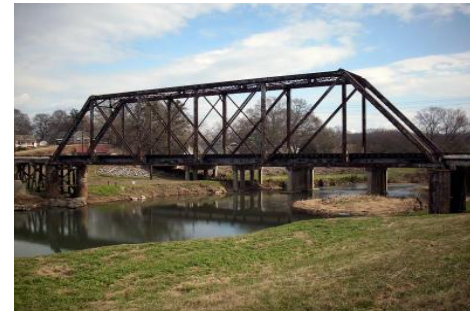
Figure 87: Chattooga River Railroad bridge. Trion, GA.
