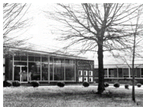
Figure 86: Historic Photo of Chattooga County Hospital in Summerville, GA which opened in 1951. Photo courtesy of Chattooga County Historic Society
