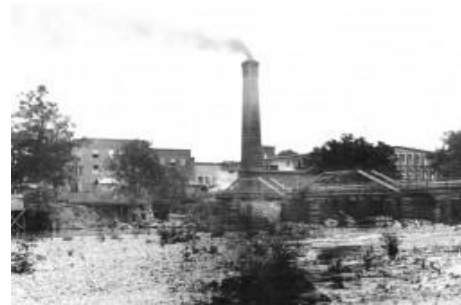
Figure 21: Historic photo of Trion Mill 1895. Photo courtesy of the Chattooga County Historical Society
