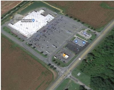
Figure 46: Walmart shopping center located between Summerville and Trion off of Hwy 27
