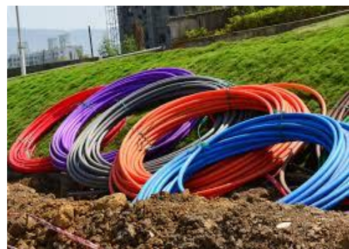
Figure 57: In the age of wireless connectivity, invisible to the naked eye, costly physical infrastructure is required to provide reliable, high - speed broadband. The infrastructure primarily consists of buried fiber optic cable as shown above
