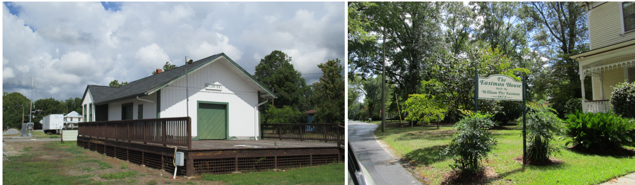
L Historic Railway Depot, Milan R Historic Residence, Eastman
