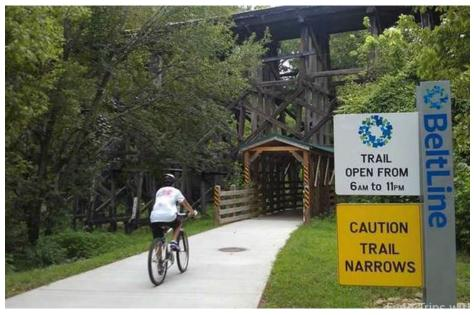
Canopy protective structure over trail when going under rail roads.
