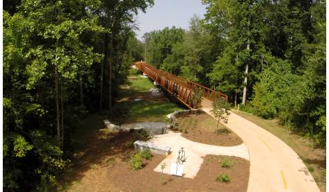
Prefabricated steel bridges allow trails to cross above existing roads and waterways.
