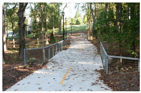
Custom steel bridge with handrail to span existing drainage swale.
