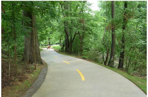
Sloping trail <u>away</u> from nearby creek into a gravel drain allows runoff to infiltrate under trail prior to entering creek.
