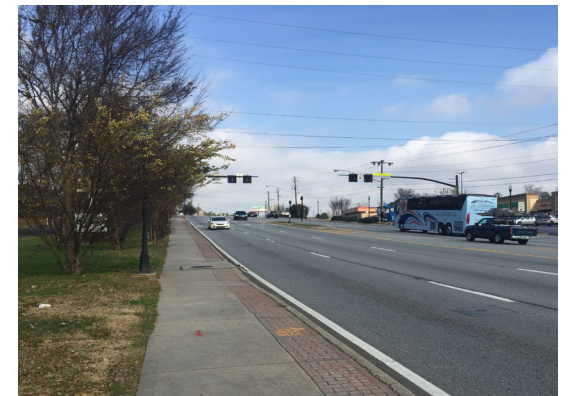
Existing pedestrian facilities along Buford Highway
