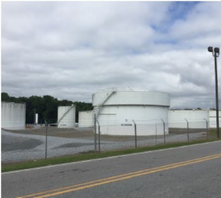
Tank farm Doraville
