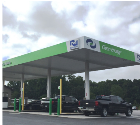
Clean energy station Doraville
