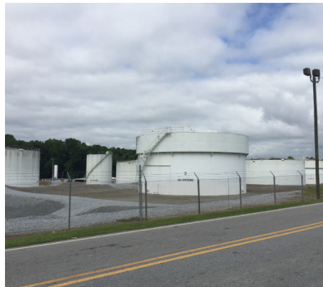
Tank farm Doraville
