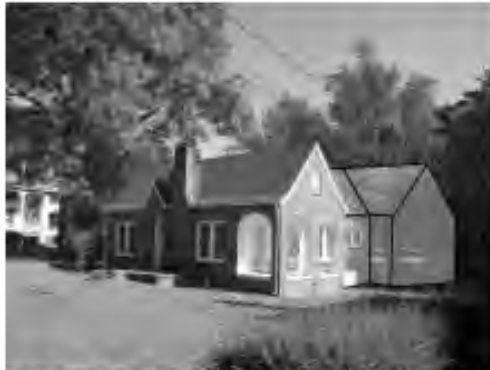
The proposed addition to this building is placed on the rear elevation, is clearly differentiated from the original structure, and is appropriately scaled.
