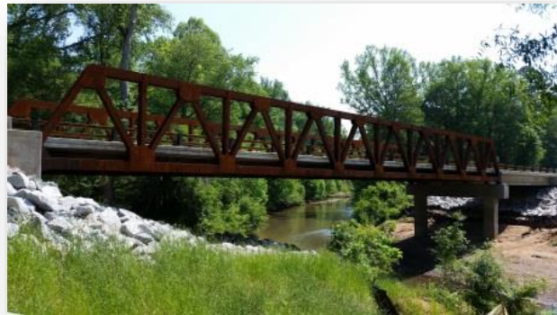
Salem Road Bridge
