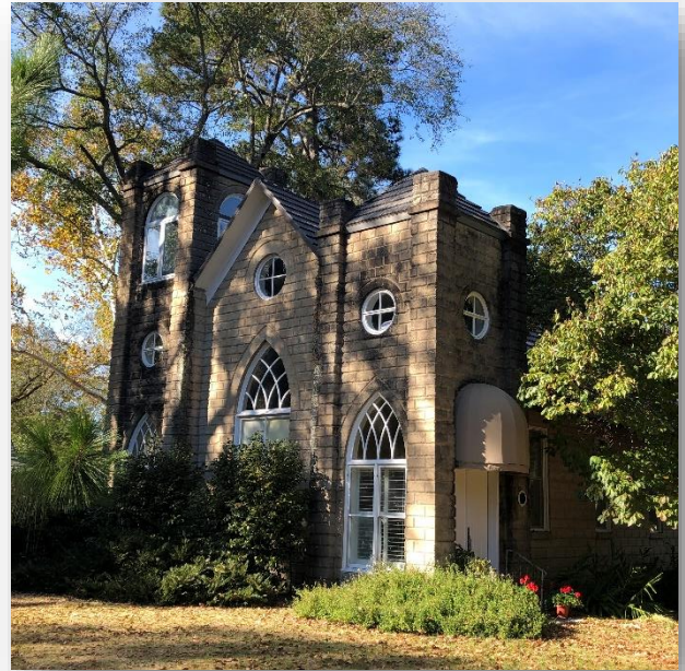
Historic Church Adaptive Reuse
