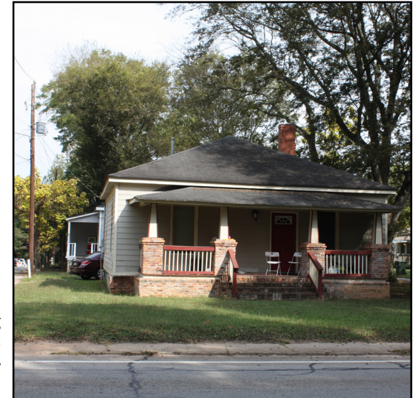
Restoration of existing buildings will continue to be a high priority for the City.
