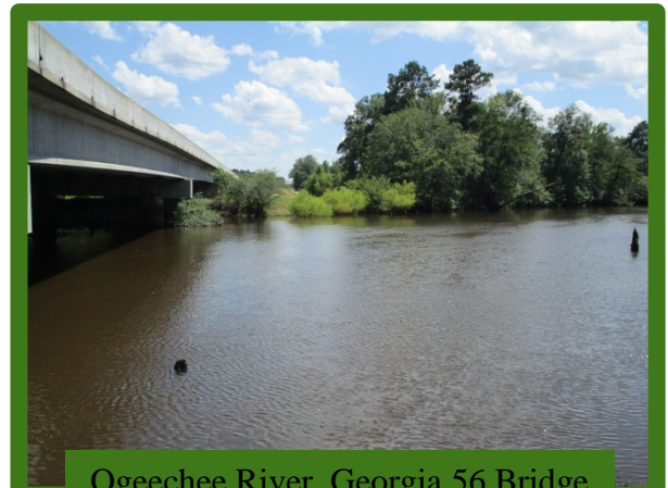
Ogeechee River, Georgia 56 Bridge
