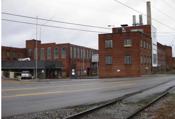
Old mill complex in redevelopment area
