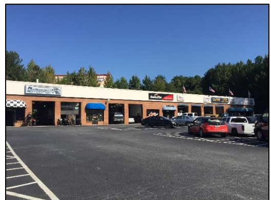
Vehicle Repair Businesses Along South 120
