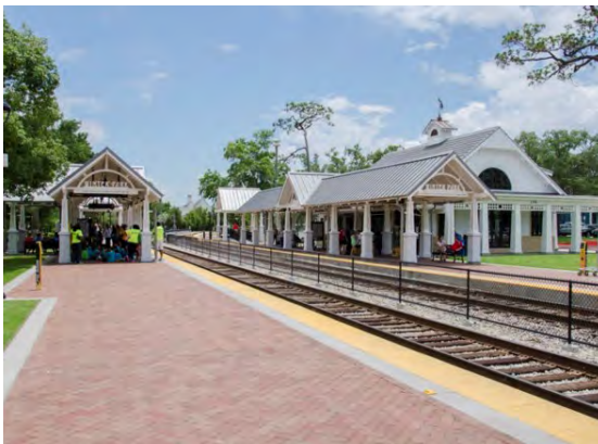
Figure 8.5d: Example Commuter Rail Station
