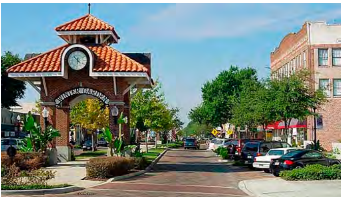
From top to bottom; 1) Streetscape project (Source: Franklin Downtown Partnership); 2) Intelligent Transportation Systems (Source: TransCore); 3) Trail connects recreational riders to Downtown Winter Garden (Source: SW Orlando Blog)
