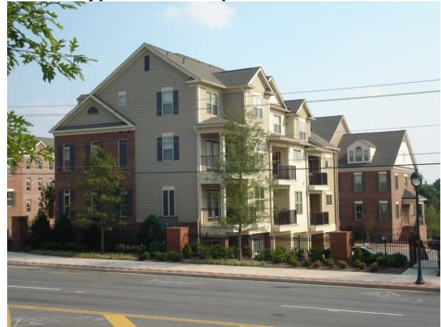
Apartments with Good Articulation of Buildings
