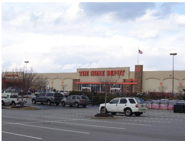
The Home Depot is representative of the growth in retail trade in the city.
