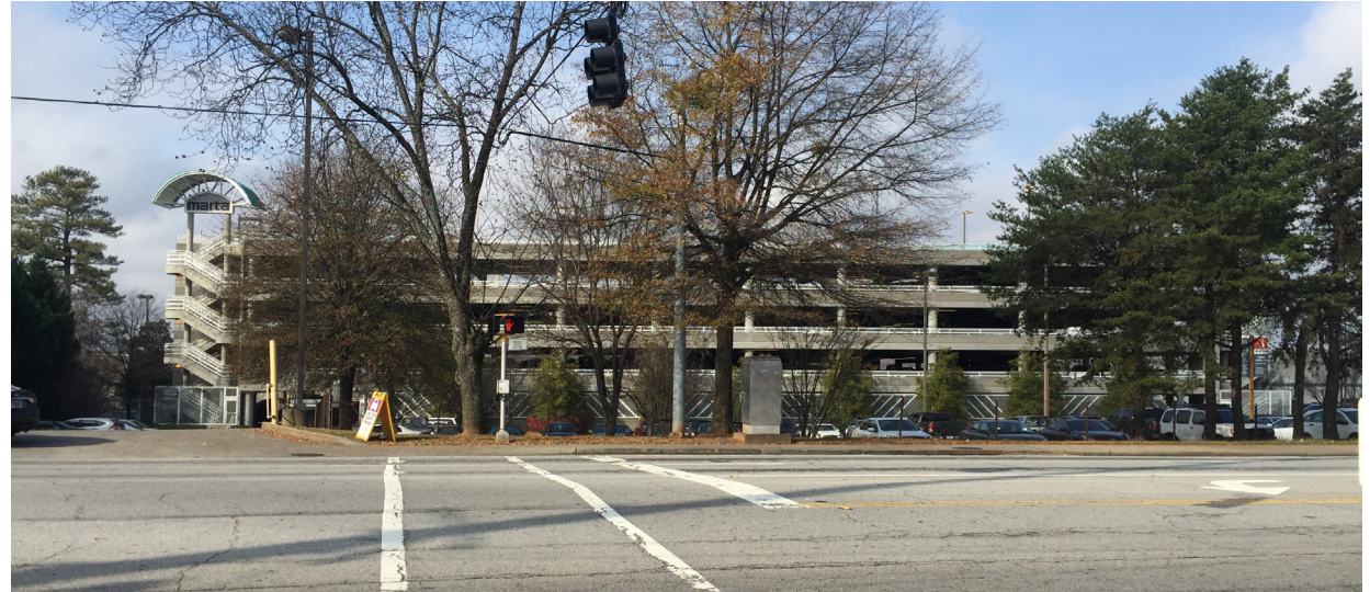
Decked parking at the Doraville MARTA station from New Peachtree Road
