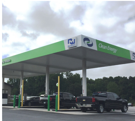
Clean energy station Doraville
