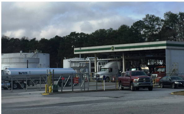
Tank farm facilities near the railroad tracks
