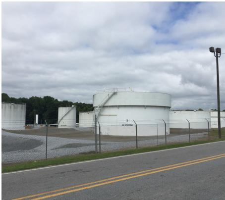
Tank farm Doraville
