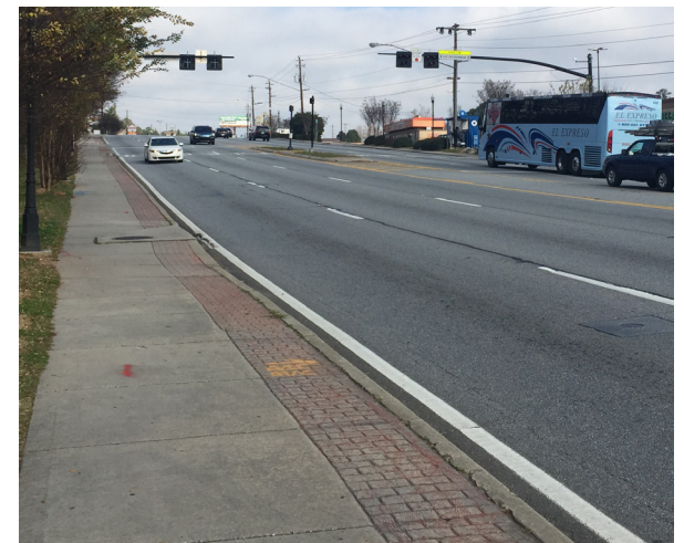
Existing pedestrian facilities along Buford Highway
