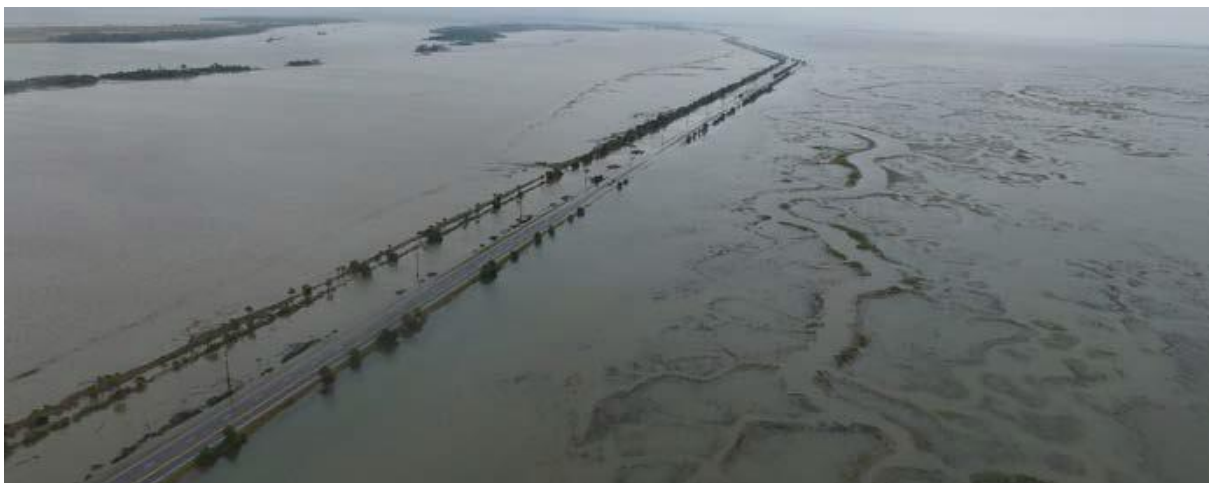
Figure 9: Flooding on U.S. Highway 80 during a King Tide Event in October 2015 (Credit: Tybee Island Police Department)
