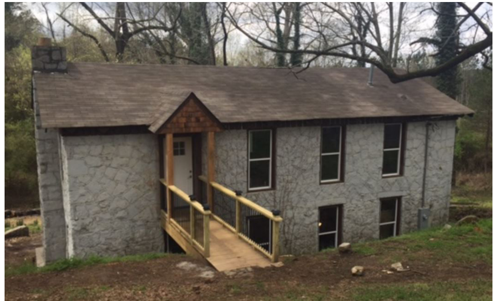
The former dormitory shown above and the boy scout hut shown below are being repurposed for institutional or community uses in Porterdale.
