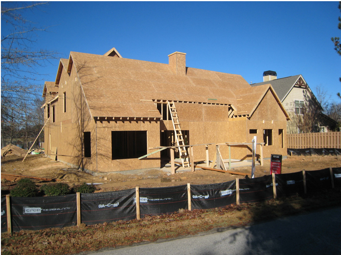
New residential construction in Newnan
