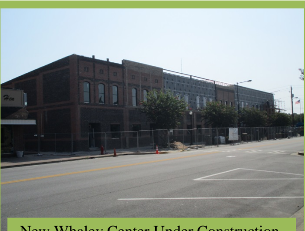
New Whaley Center Under Construction, Downtown Jesup
