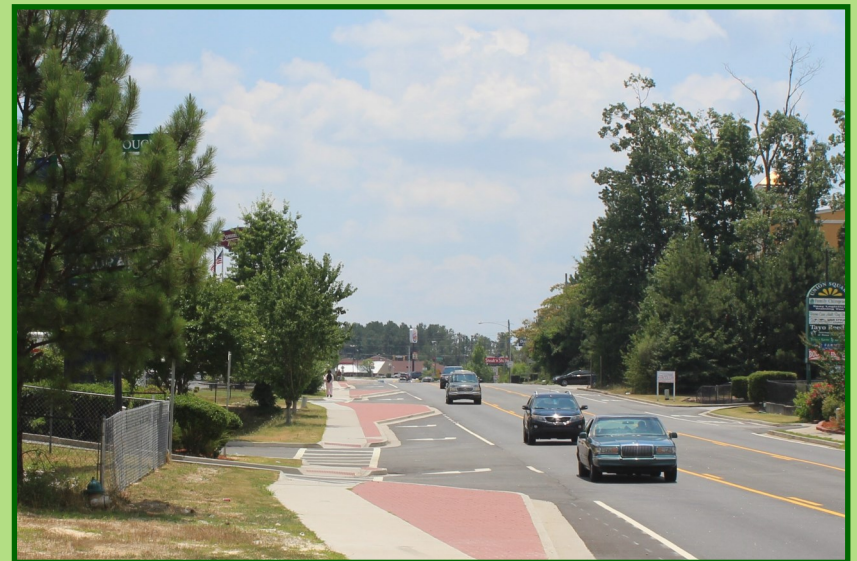
New sidewalks along Shannon Parkway
