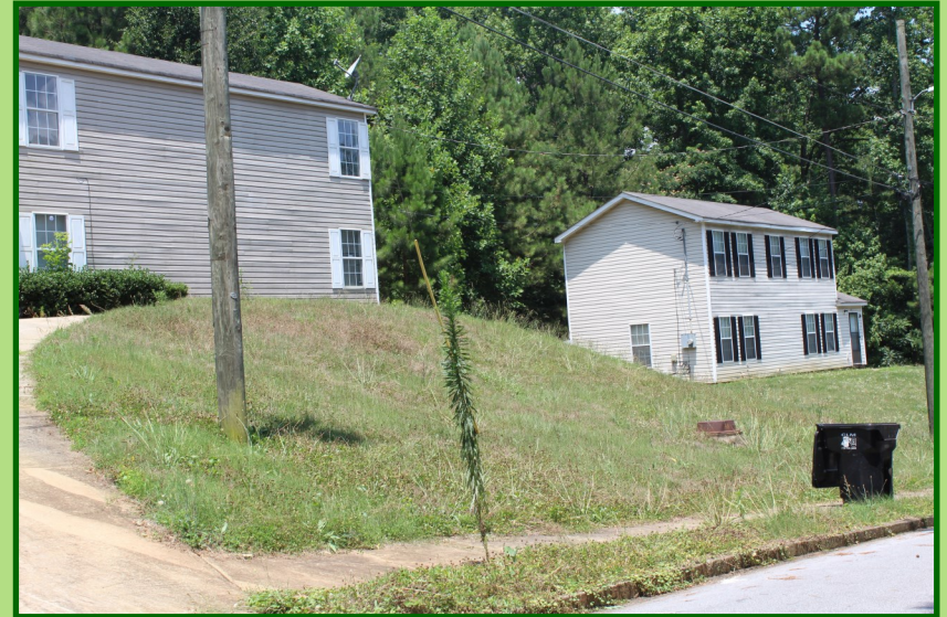
Homes off of Lower Dixie Lake Road.
