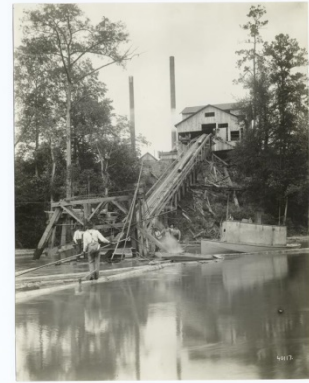
Historic Ocmulgee River Lumber Company Log Slide, Lumber City
