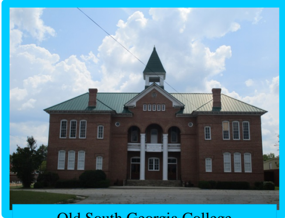
Old South Georgia College (Telfair Center for the Arts), McRae-Helena
