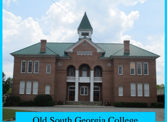
Old South Georgia College (Telfair Center for the Arts)
