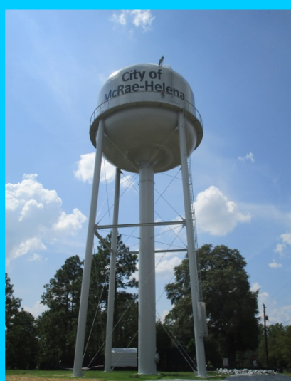
New McRae-Helena Water Tower
