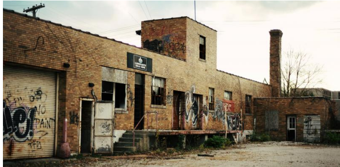
Example of a Brownfield
