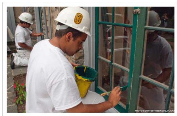
Workers Restoring Historic Windows
