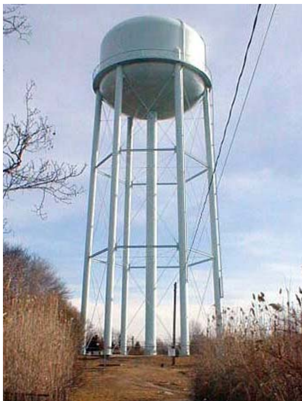
Example of a water tower
