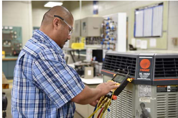
Technical College student learning HVAC repair
