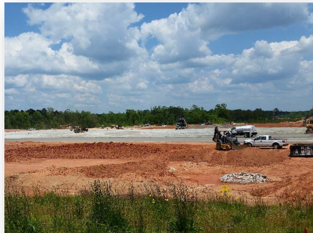
FIGURE 29: CONSTRUCTION SITE OF GLOVIS' NEW LOCAL LOCATION
