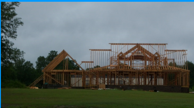
House under Construction along Georgia 15
