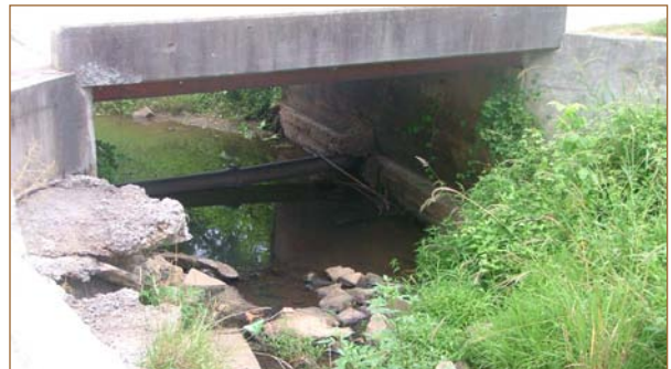
Small creek along Lyndon Avenue
