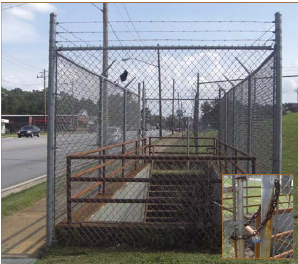
Pedestrian Underpass, N Expressway (US 19/41)
