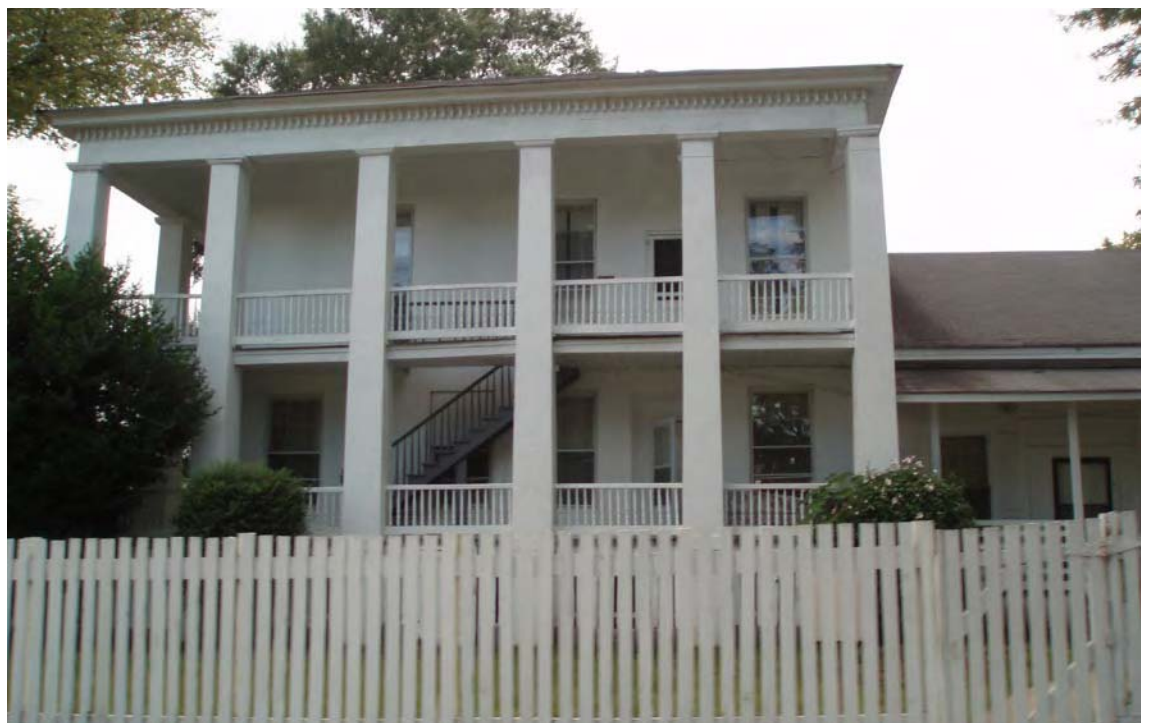
Figure 48: Griffin Medical College building
