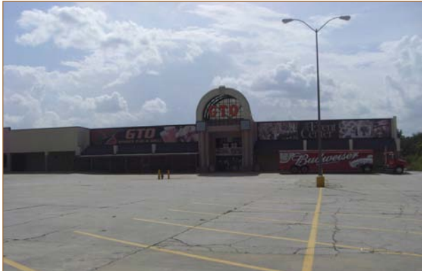
Expansive parking under utilized; void of landscape or pedestrian connectivity with site services or surrounding land uses.
