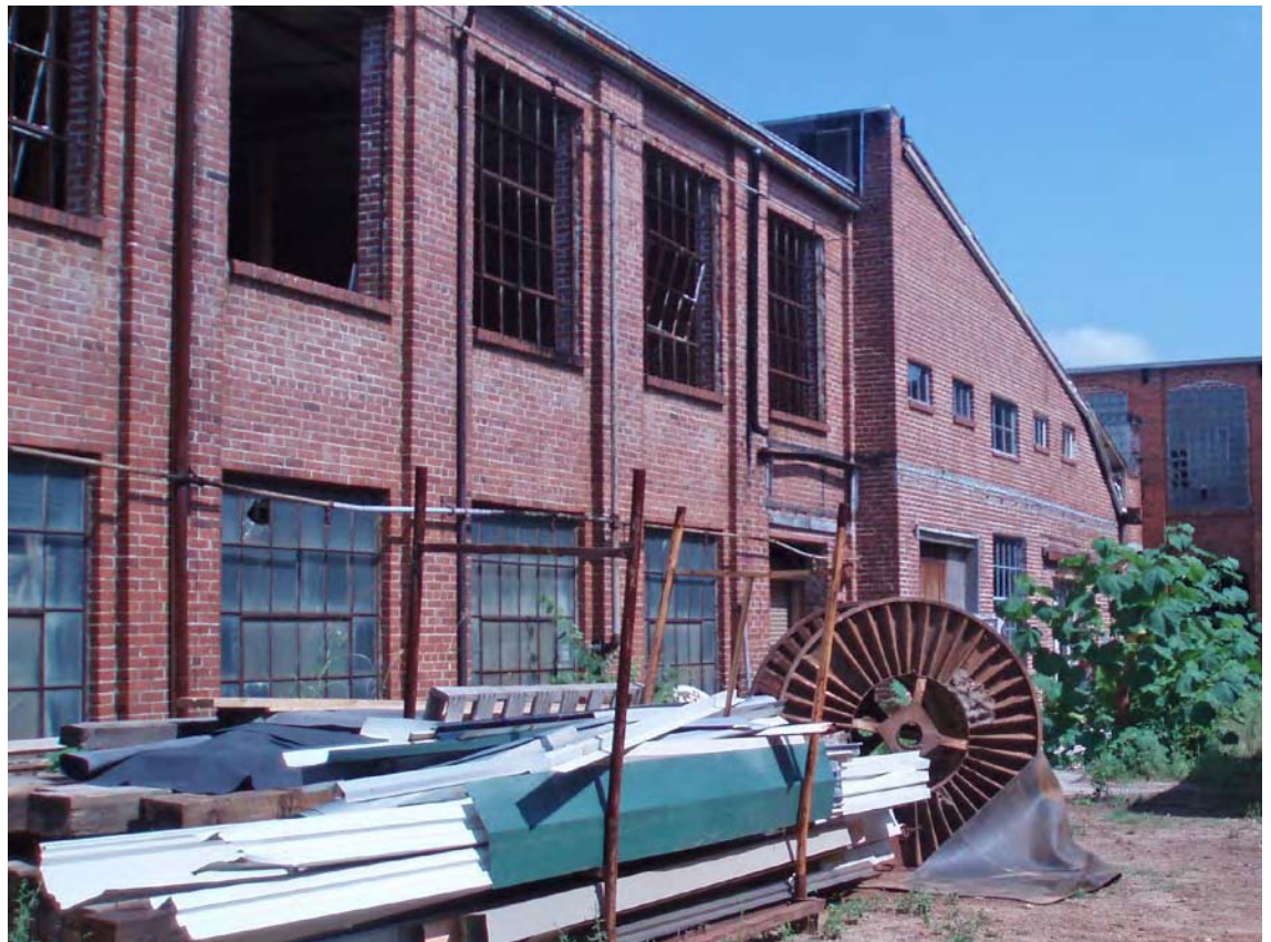
Figure 6: Plentiful Historic Rehabilitation Opportunities
