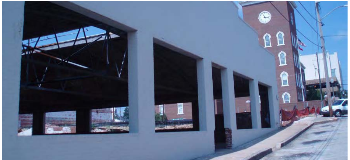
Figure 32: Conference Center building rehabilitation
