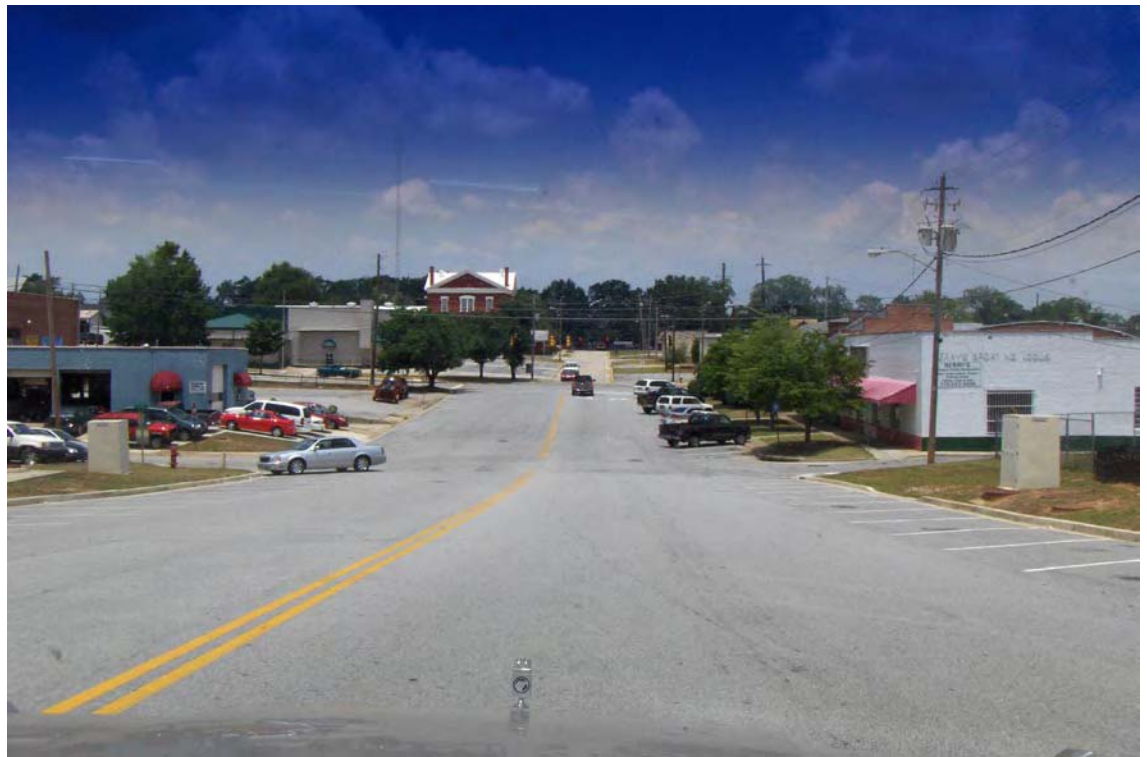
Figure 61: Existing wide right-of- way at Fifth Street
