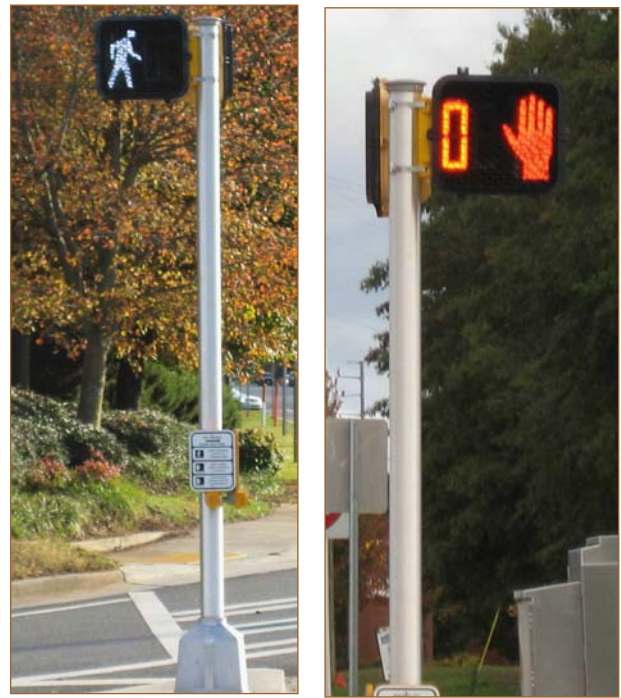
Install pedestrian countdown signals to improve pedestrian safety
