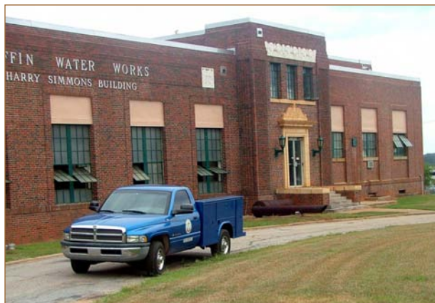
Griffin's Water Treatment Facility on North Expressway
