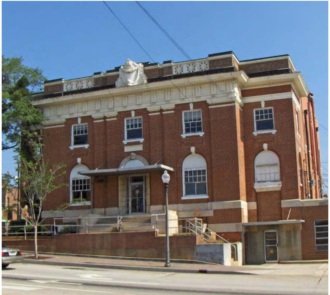
Figure 7: Historic City Hall, currently vacant
