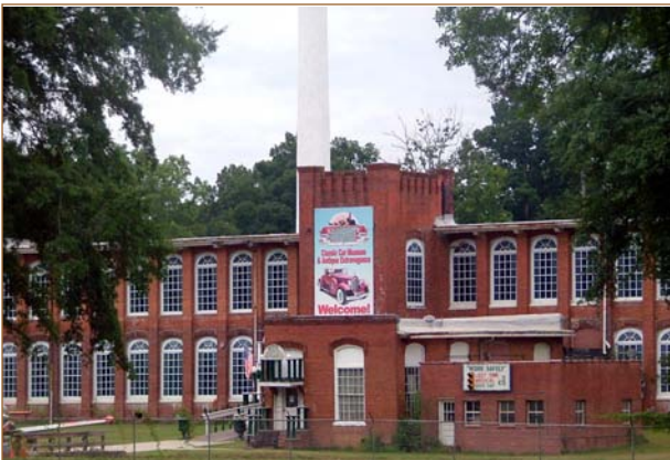
Rushton Mills Redevelopment on Lyndon Avenue
