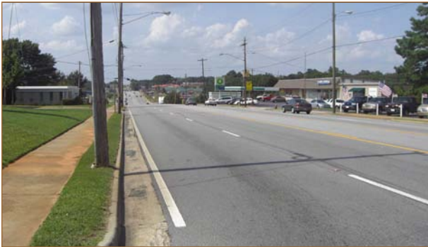
Existing condition of N Expressway
