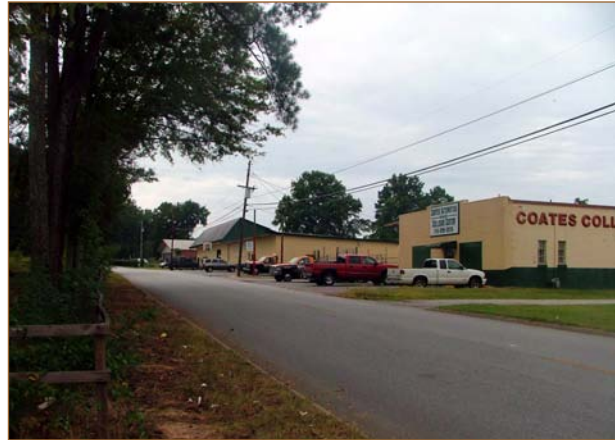
Lack of transition buffer from commercial to residential land uses. Lackluster streetscape include overhead utilities and store front parking.
