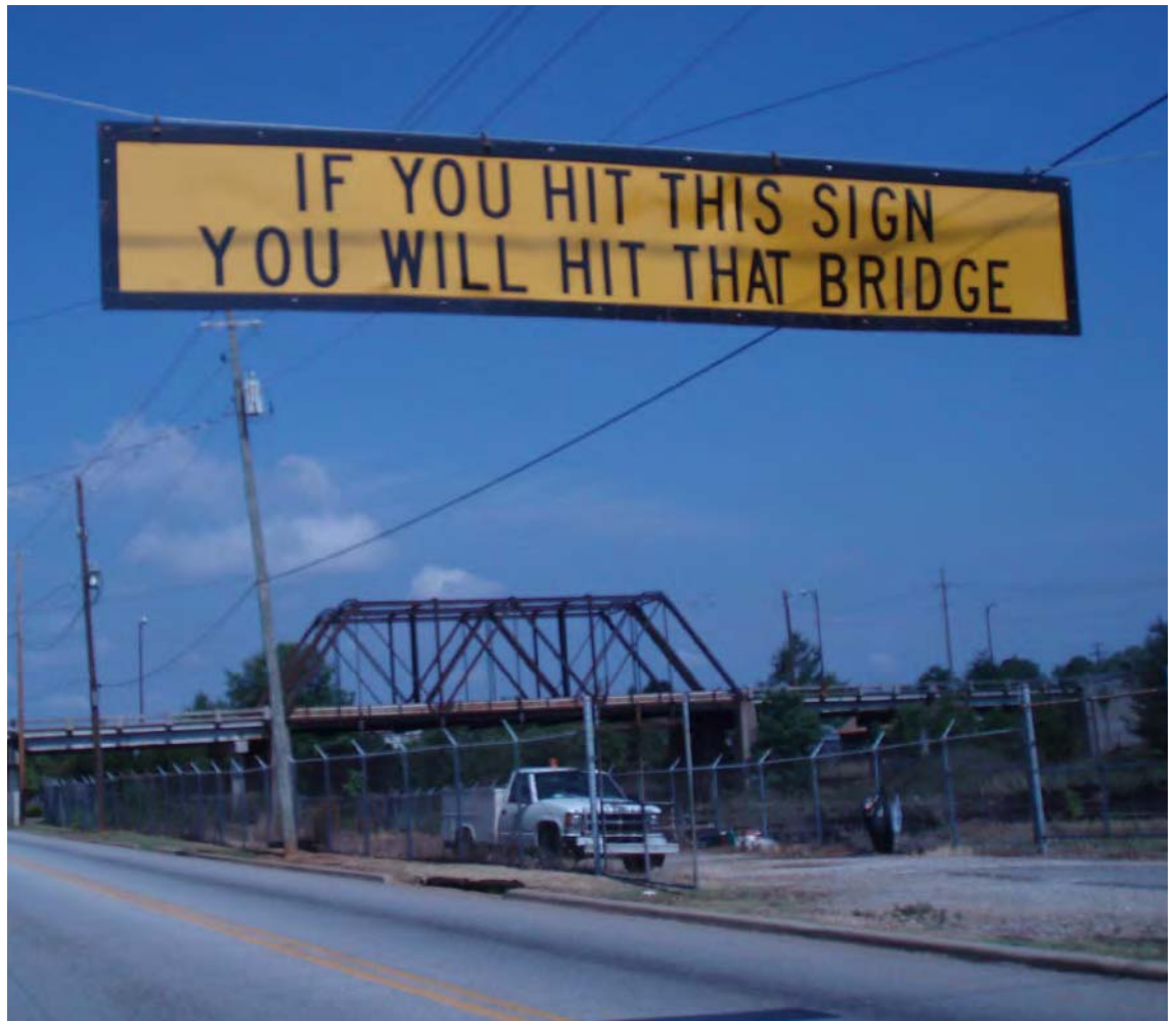
Figure 22: Warning sign for 6th Street Bridge
