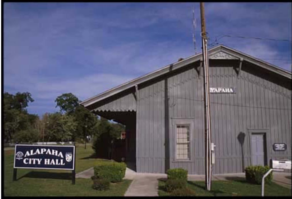
The 1881 Brunswick & Albany Railroad depot at Alapaha now serves as city hall in this Berrien County town.
