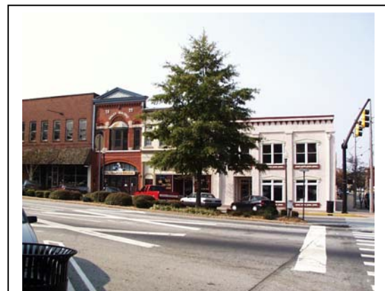
Commercial buildings and landscaped median along Hill Street
