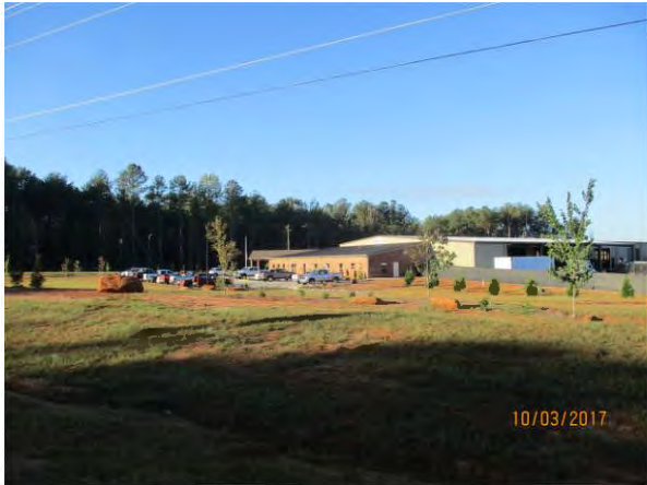
Arterial Overlay Corridor – Highway 41
