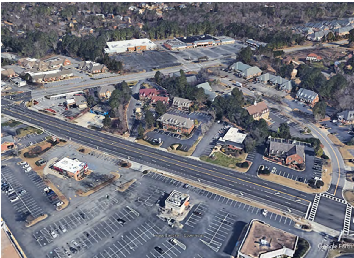
Holcomb Bridge Road – multiple access points with no deceleration lane.
