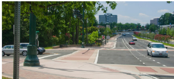
The future Holcomb Bridge Corridor will include pedestrian facilities like the ones shown at left so pedestrians can walk and cross safely.
