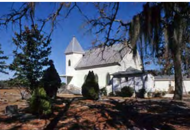
McCanaan Missionary Baptist Church and Cemetery, located in Sardis, Burke County, was listed in the National Register in 2001. Churches comprise two-thirds of African American community landmark buildings.
