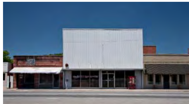
This modern style commercial building in Summerville, Chattooga County, is an example of the mid-20th-century updating of older buildings with new, modern facades.
