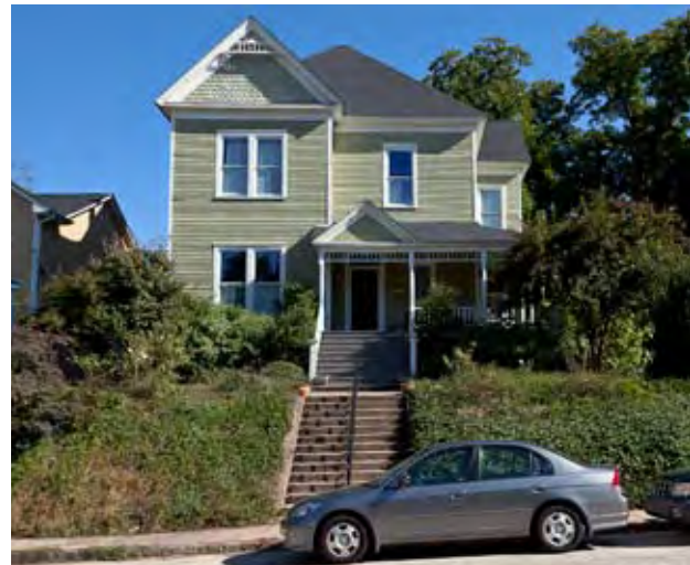
Historic house on Adams Street, Macon, Bibb County, after rehabilitation using the historic preservation tax incentives.
