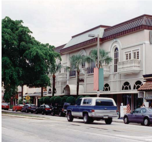
Figure 2.6 Buildings adjacent to the sidewalk enliven a corridor
