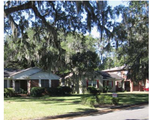
Figure 2.22 Single-family housing typical of South End Brunswick
