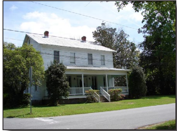
Residence located in Old Pooler Downtown
