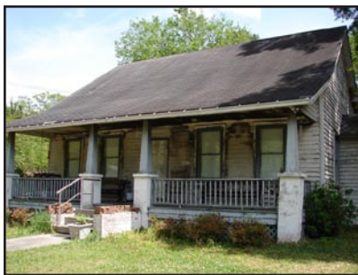
Area in need of redevelopment
