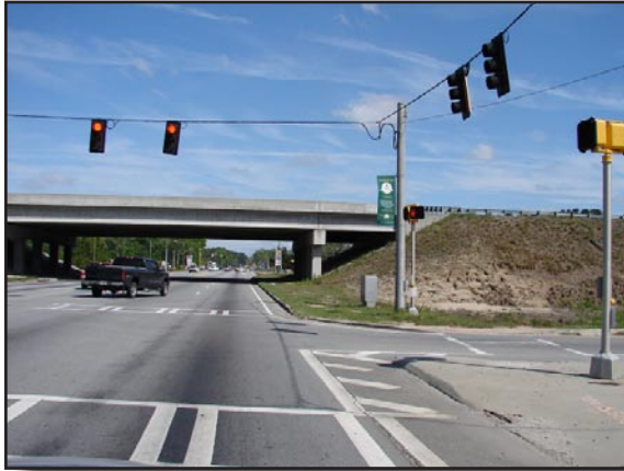
US Highway 80 - Major corridor into Downtown Pooler
