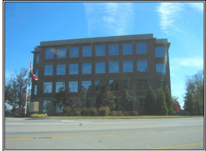
Commercial office building located in the Commercial Node
