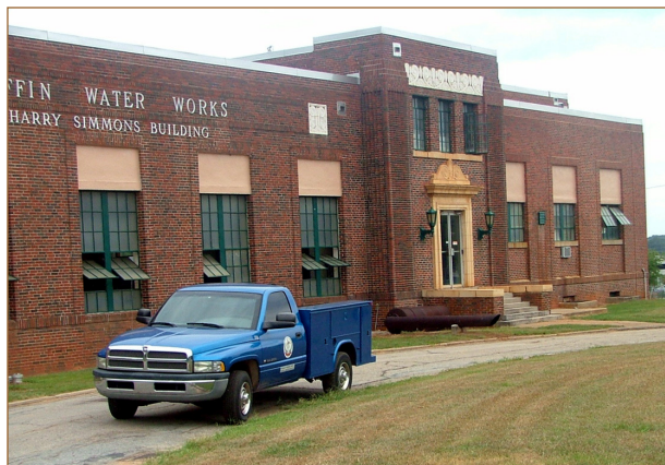
Griffin's Water Treatment Facility on North Expressway
