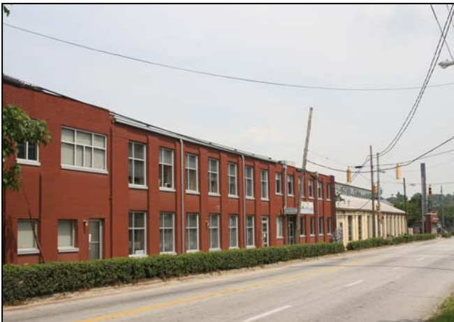
Example of Mill Adaptive Reuse: Puritan Mill Complex: Atlanta, Ga
