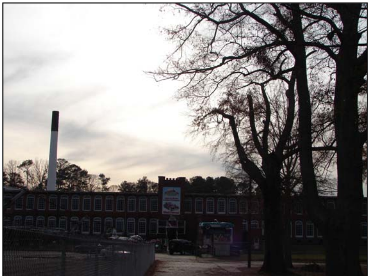
Rushton Mill Building and Site
