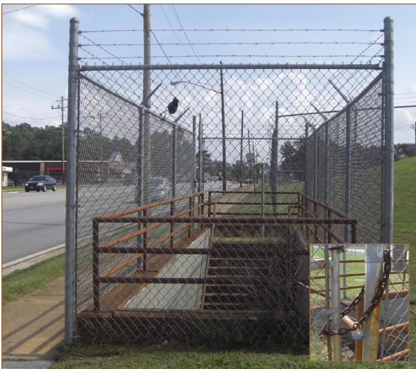
Pedestrian Underpass, N Expressway (US 19/41)
