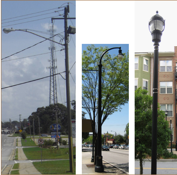
Replacing existing roadway lighting with ornamental roadway lighting
