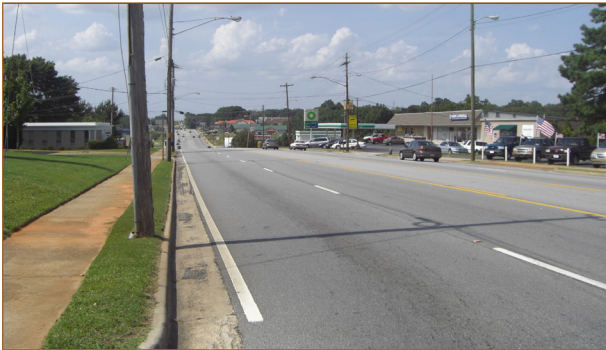
Existing condition of N Expressway
