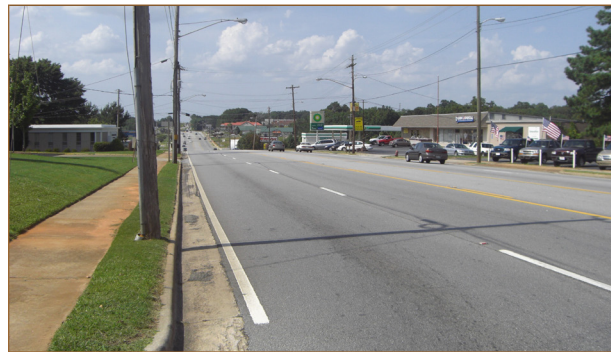
Existing condition of N Expressway (US 19/41)
