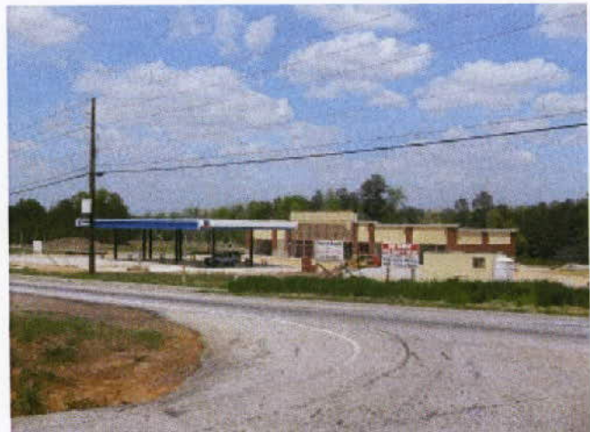
Commercial Development Under Construction, Sigman Road
