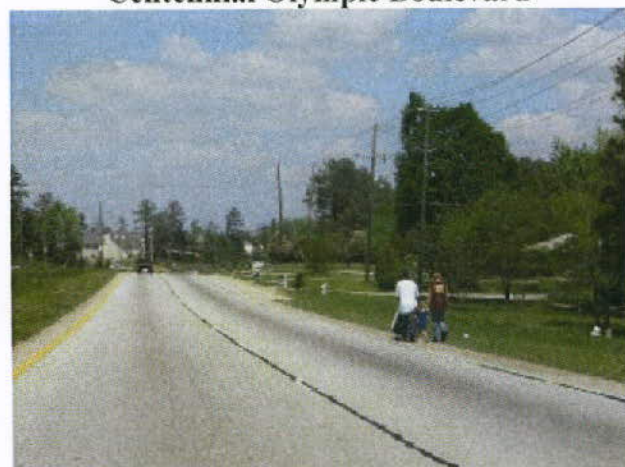
Pedestrians with Narrow Sidewalk Perilously Close to Travel Way
