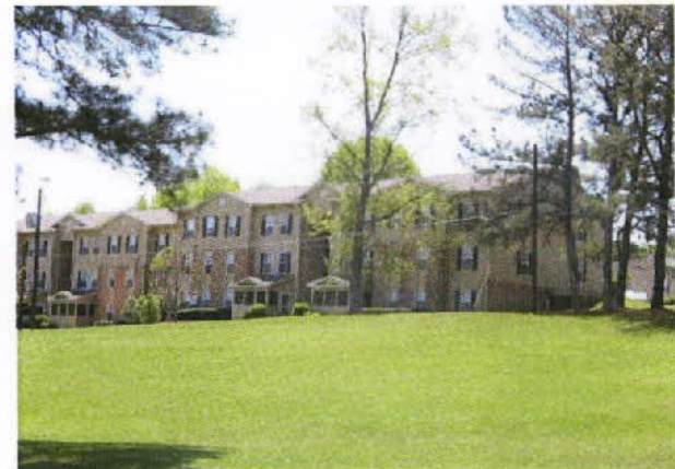
Apartments Along Pine Log Road
