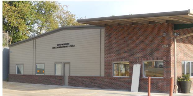
New City of Norcross Public Works Building Relocated from Downtown to Lively St.
