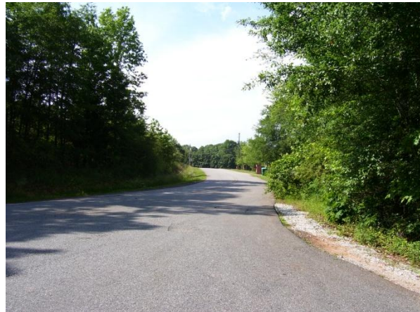
Representative street conditions in large lot-rural character area.
