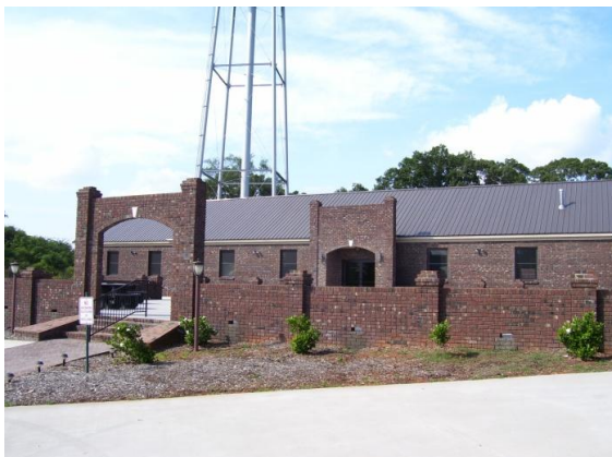
Nicholson's community center, along with city hall, form a government institutional complex on the north side of the Nicholson Town Center.
