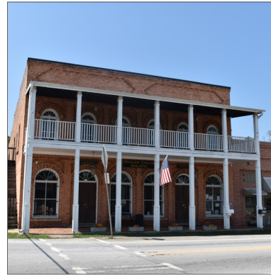
Figure 22. The Ziegler-Childs Building
