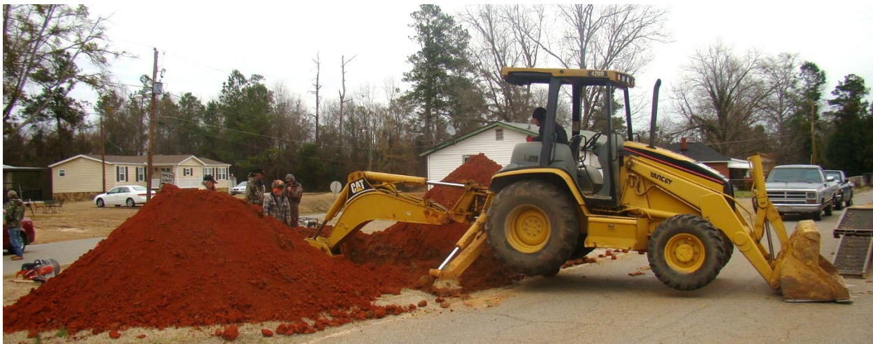
Photo 1: Utility repairs in the City of Jeffersonville (MGRC Staff Photo)
