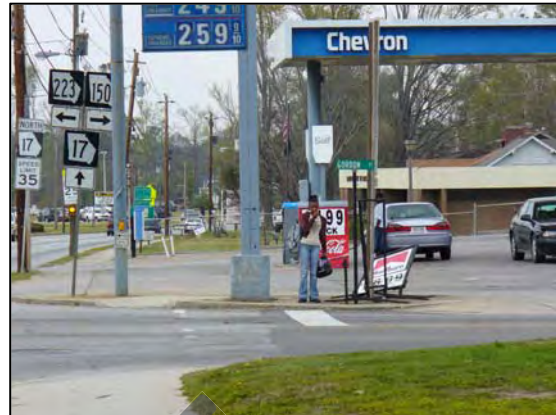
Faded crosswalk along Main Street
