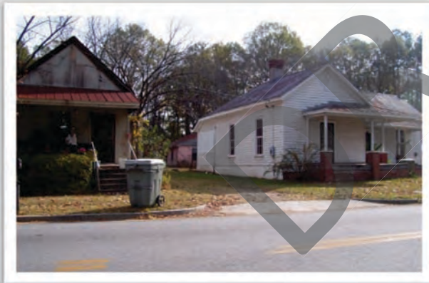
Dilapidated housing stock and a lack of positive identity define the character of the TN-D character area
