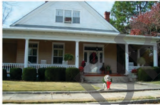
A typical well maintained older home in the TN-S character area the front porch and sidewalks contribute to the character of the neighborhood
