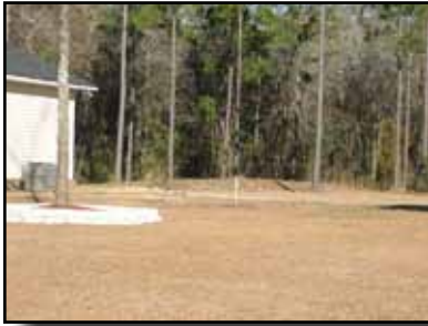
Septic Tank Mound
