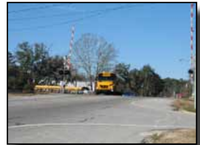
Highway 57 Railroad Crossing in Ludowici
