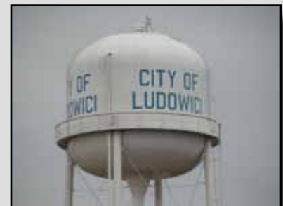
Water Tank at Industrial Park
