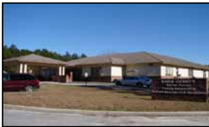
Multi Use Social Services Facility
