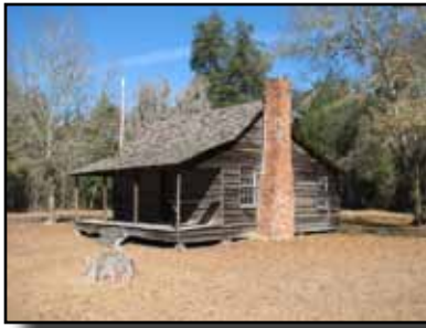
Early House at Jones Creek Community Park
