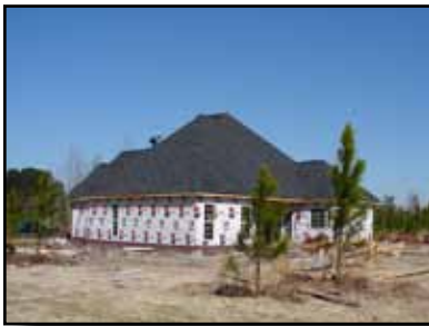
New House Construction
