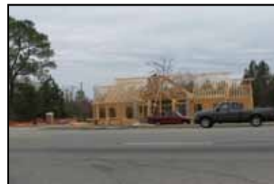
New Business Construction
