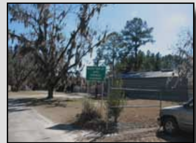
Road Maintenance Facility
