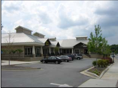
Mixed office and retail development.
