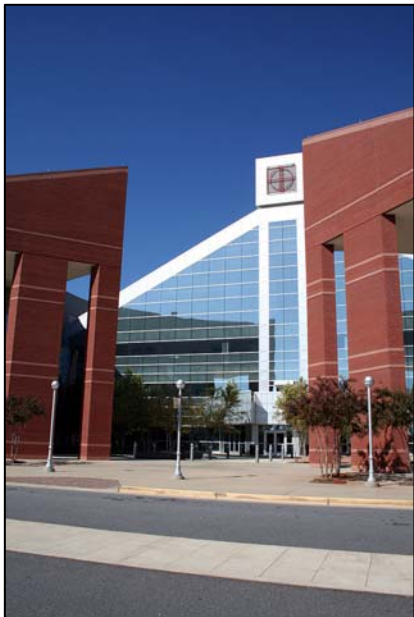
Georgia Gwinnett College's Administration Building.
