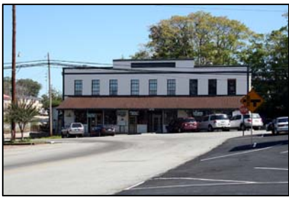
Historic Building in the Depot area.
