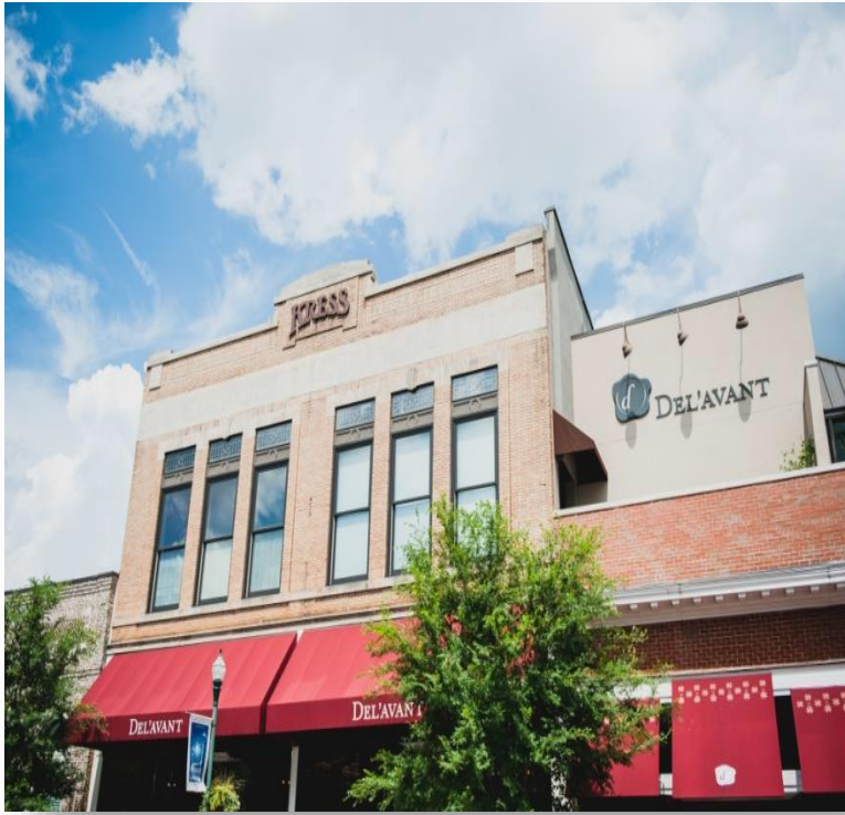
Figure 2: Historic Kress Building. Now Del'Avant Event Center
