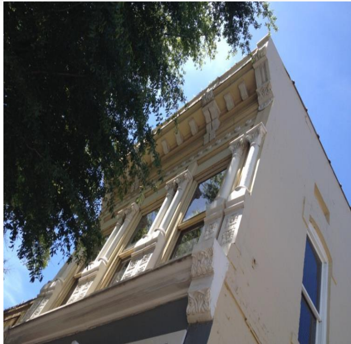
Figure 3: Downtown building containing historic metal facade.
