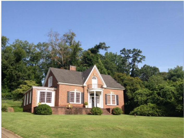
Figure 4: Traditional home in LaGrange
