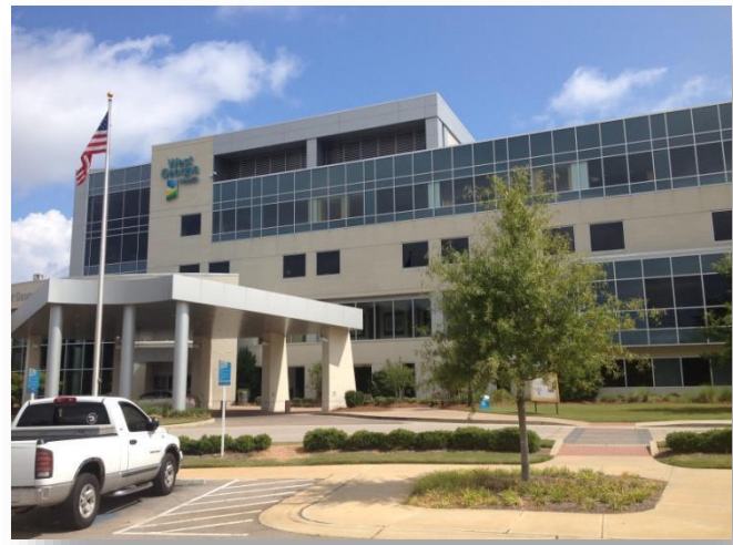
Figure 19: West Georgia Medical Center
