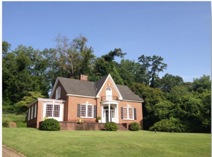
Figure 4: Traditional home in LaGrange
