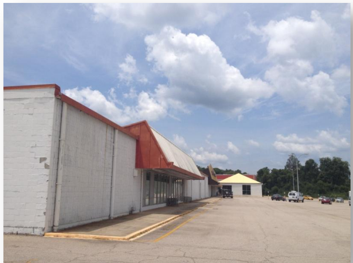
Figure 14: Commerce Avenue strip center
