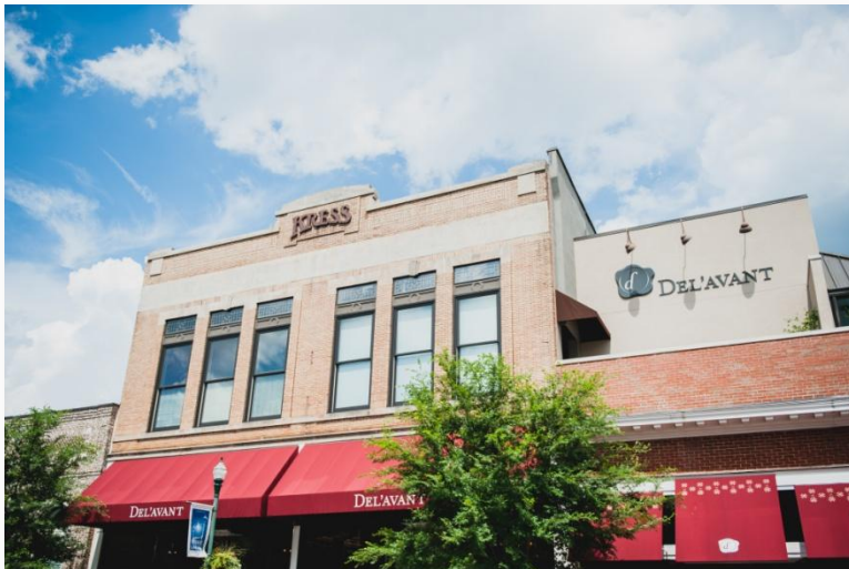
Figure 2: Historic Kress Building. Now Del'Avant Event Center
